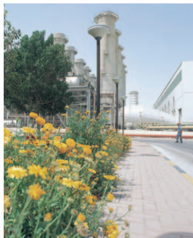
When Alba was founded, annual production capacity was to be 56,000 mt, but right away this figure was raised to 120,000 mt. Today, it stands at over 870,000 mt
