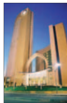
The Corinthian Hotel in Tripoli, a five-star Libyan-Maltese joint venture
