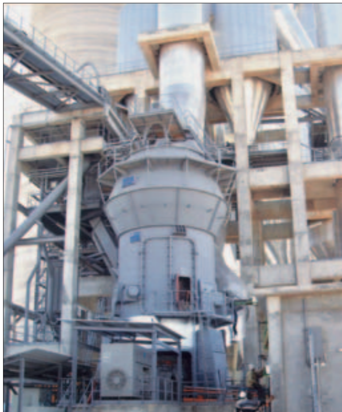
Production has already started at AUCC's new cement plant where it will eventually reach more than 3 million tpa.
