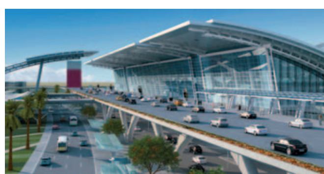
The first phase of the New Doha International Airport (NDIA) is scheduled for completion by the end of this year and will have an annual capacity of 24 million passengers
