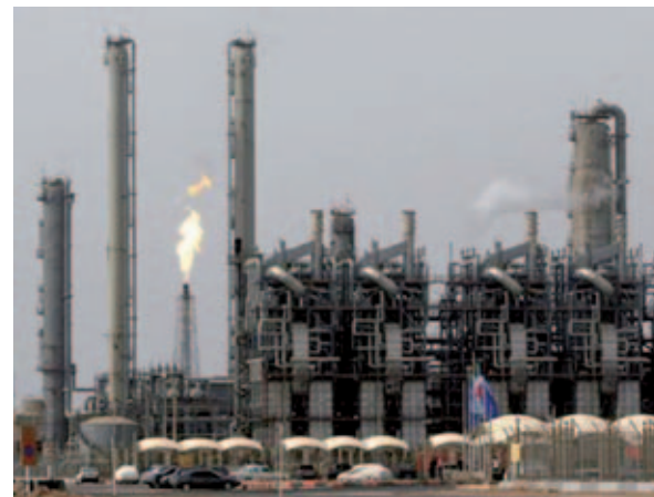
The Q-Chem plant is operated by QP and Chevron Phillips
