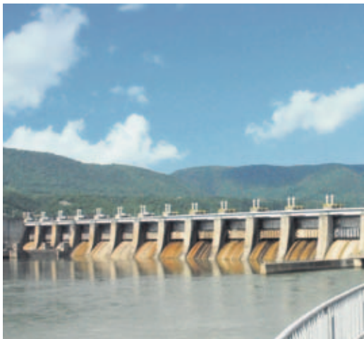
The power generator's new Hidroenergetica entity is designed to maximize a mix of energy sources
