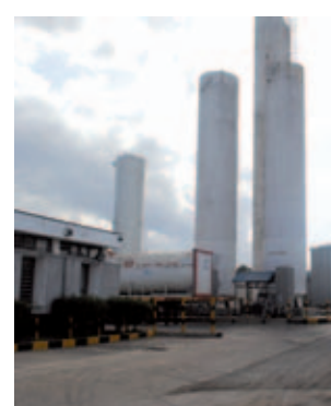
TOL Gases has three production sites located in Dar es Salaam
